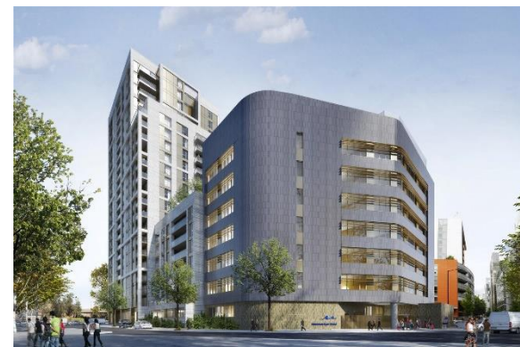
£104m Dudley House – mixed-use development
