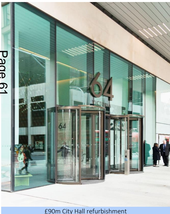
£90m City Hall refurbishment
